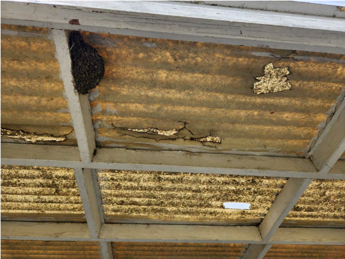
Clean shelters and replace roofs
