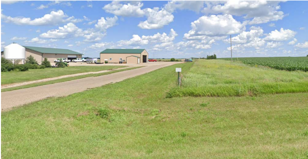
Menoken Farm Facility
