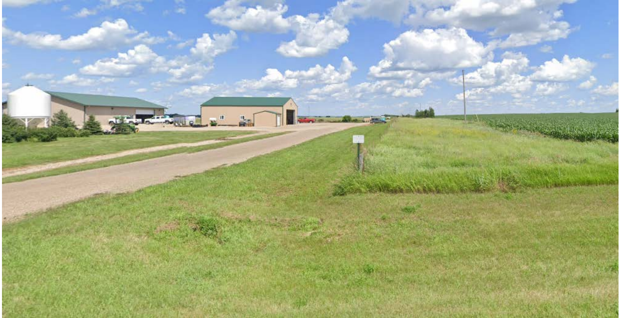
Menoken Farm Facility
